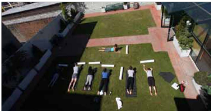
Yoga students work out on Green Fitness Studio's living roof that acts as natural insulation for the Brooklyn, N.Y., facility. Photo courtesy of Green Fitness Studio
